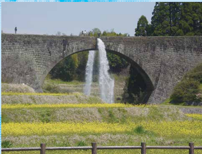
Water is discharged from the center of the Tsujun Bridge at scheduled times throughout the year.
